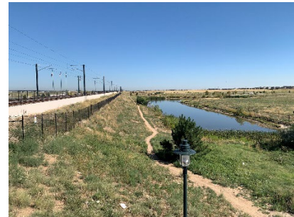
Social trail highlighting lack of connectivity at 40th & Airport Boulevard Station
