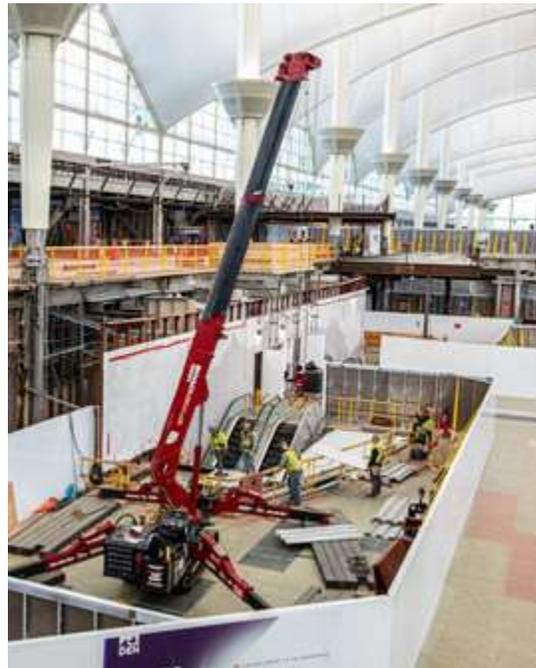
In the coming weeks, demolition should be completed, and a large crane will be set up curbside on Level 6 to install structural steel at the perimeter of the terminal, where the new restrooms will be located.
