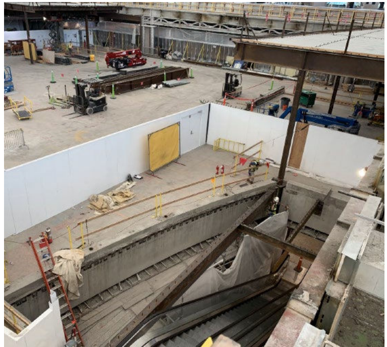
GREAT HALL CONSTRUCTION IN PROGRESS | Sections of Denver International Airport's main terminal were demolished as part of the Great Hall renovations — specifically, the center exterior terminal (at left) and the arrival escalators for the airport's underground passenger train (above). PHOTOS BY DENVER INTERNATIONAL AIRPORT STAFF
