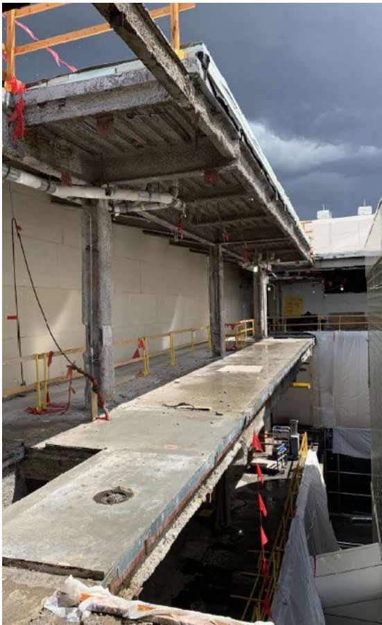
GREAT HALL CONSTRUCTION IN PROGRESS | Sections of Denver International Airport's main terminal were demolished as part of the Great Hall renovations — specifically, the center exterior terminal (at left) and the arrival escalators for the airport's underground passenger train (above). PHOTOS BY DENVER INTERNATIONAL AIRPORT STAFF
